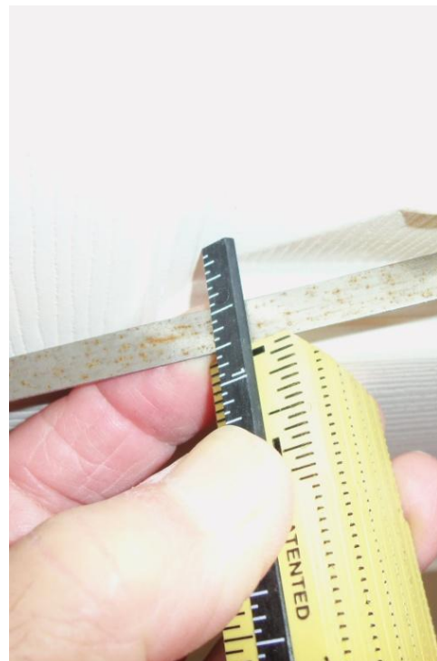
1 3/4 inch door has 7/16 inch recesses into both faces The door thickness is only 7/8 inch at the recesses.
