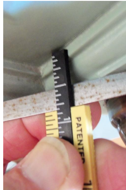
1 3/8 inch door has 1/2 inch recesses into both faces The door thickness is only 3/8 inch at the recesses.
