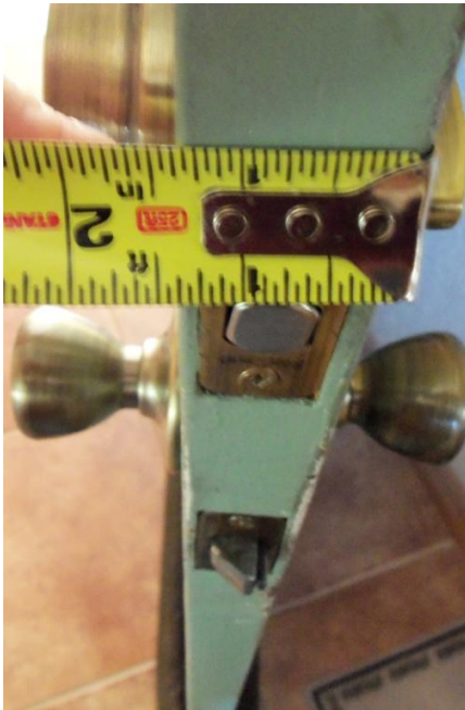
1 3/8 inch door between garage and dwelling This door is a real solid wood door.
