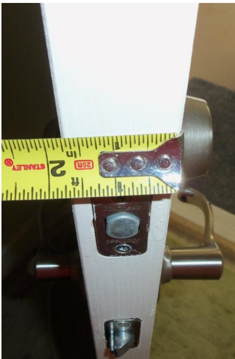
1 3/4 inch door between garage and dwelling This door is a “solid core door” with hardwood face skins.
